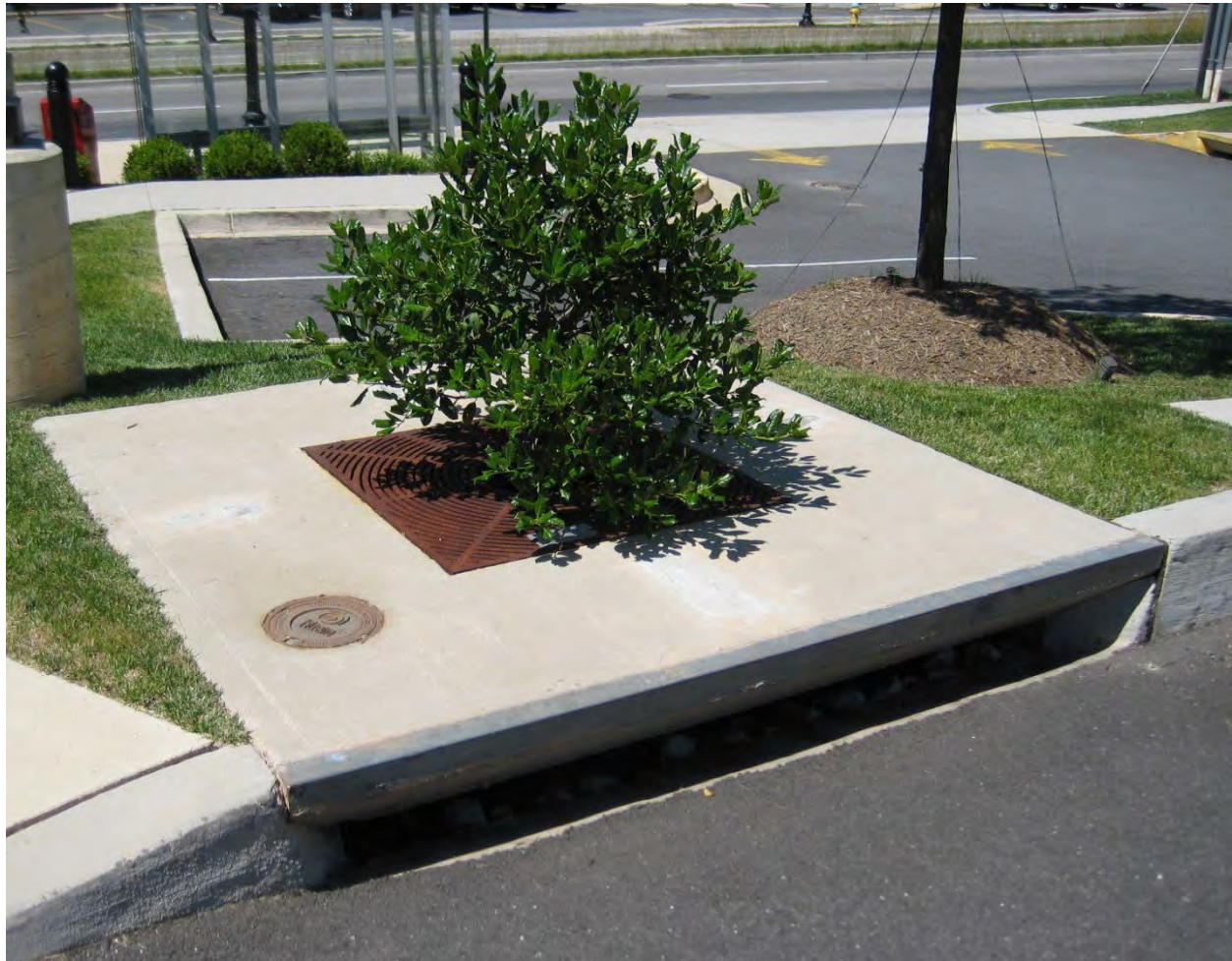
Figure 59 – Catch Basin Filtration
