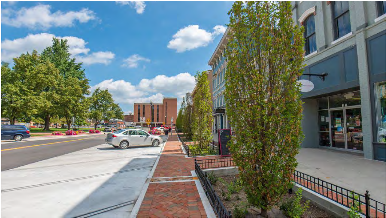
Figure 57 – Curbside Rain Gardens
