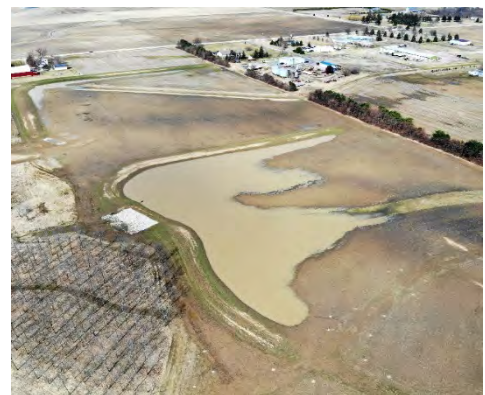
FIGURE 22: AERIAL: SAUDER VILLAGE ENGINEERED DIKES
